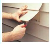
Wedge tip under the bottom end of overlapping panel and hook on the back lip of buttlock in one easy motion.
